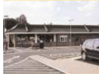
A recent installation at a fast food outlet
