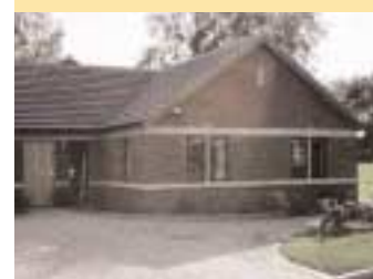
A recent installation at a housing development
